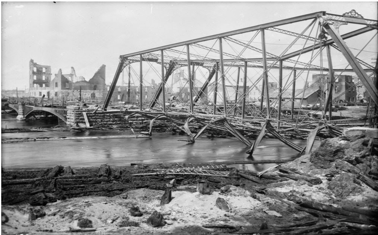
Figure 18: Chaudière Bridge taken on April 27, 1900 (photo by Horatio Needham Topley)
